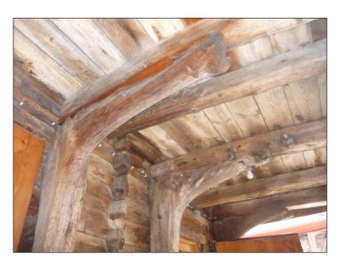
"These are tree trunks with roots attached, inverted, and used as support beams for a roof overhang in Bergen, Norway. I'd never seen anything like this done before."
